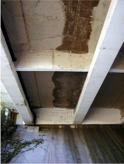
Figure 2: contamination of concrete bridge deck
