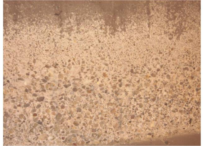
Figure 3: effect on deicing salts – scaling – on bridge concrete protection structures
