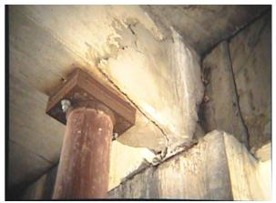
Figure 5: inefficient concrete beam repair operation (Emmons *et al.*, 1994)
