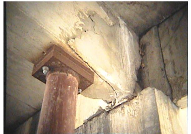
Figure 5: inefficient concrete beam repair operation (Emmons *et al.*, 1994)
