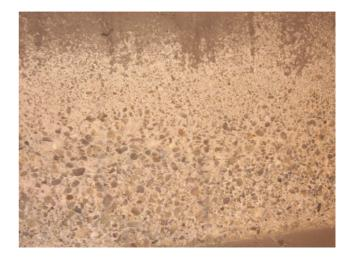
Figure 2: contamination of concrete bridge deck
