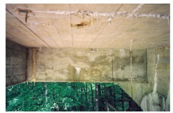
Figure 4: leakage of Ca(OH)<sub>2</sub> through cracked concrete bridge deck
