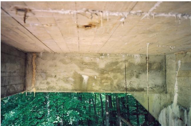
Figure 4: leakage of  $\text{Ca(OH)}_2$  through cracked concrete bridge deck
