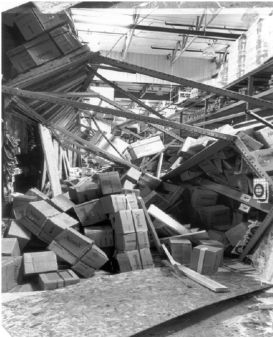
Figure 2: (a) – Collapse of a rack structure during Northridge earthquake (1994) – (b) Fall of goods during Northridge earthquake (1994) – See Ref. [4]
