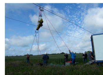
Ampacimon live line installation (220 kV) RTE network. Running system form June 2009.
