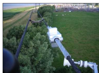
Ampacimon unit (380 kV, Doel-Zandvliet, BE) ; ELIA, running system from July 2008.
