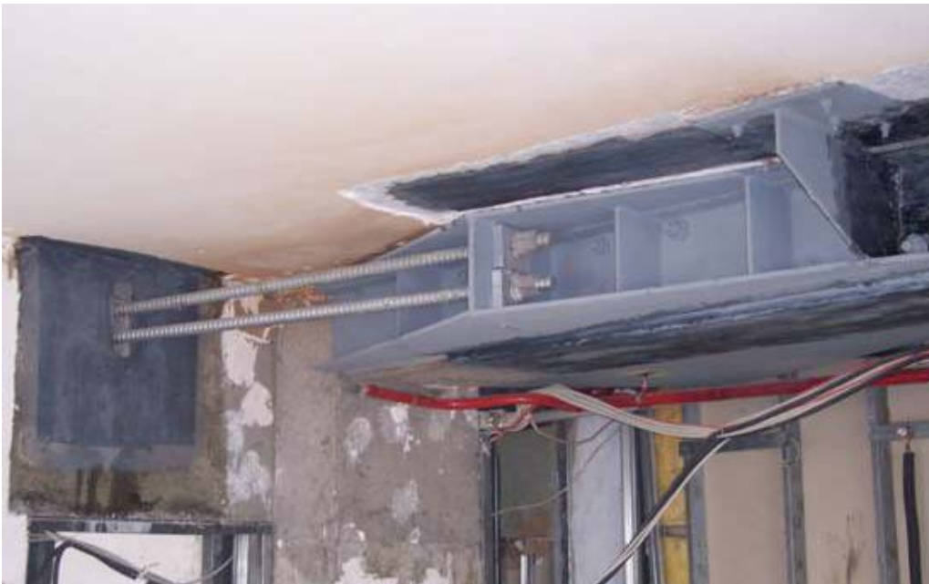
Figure 12. Rods passing through transverse beam adjacent to expansion joint.
