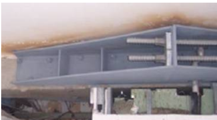
Figure 11. Connection of Dywidag rods to longitudinal beam.
