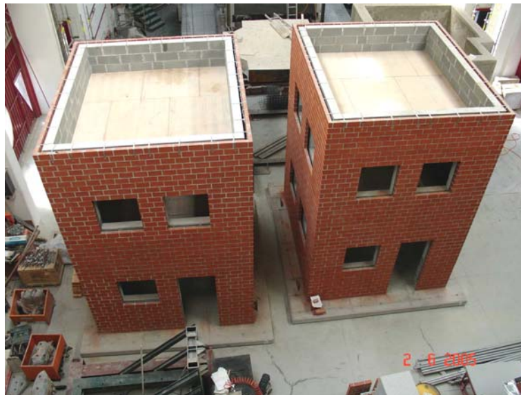
Figure 3 – The two models at the end of construction, Model 1 on the right and Model 2 (reinforced house) on the left
