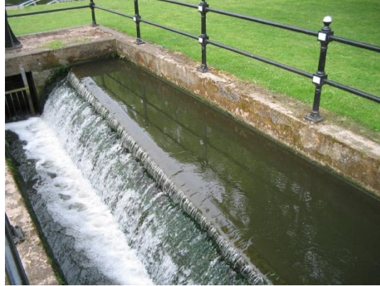
Figure II-4 Flow over a side weir
