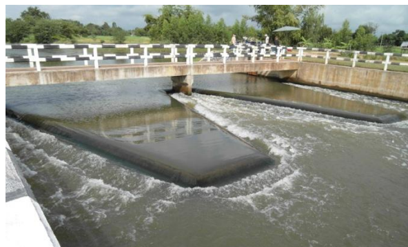
Figure II-5 Flow over a labyrinth weir
