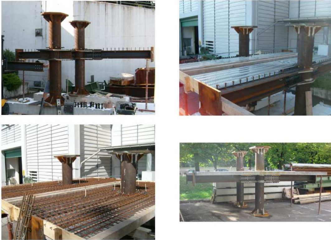
Figure 40. Realization of beam-to-column joints at the UNITN Laboratory
