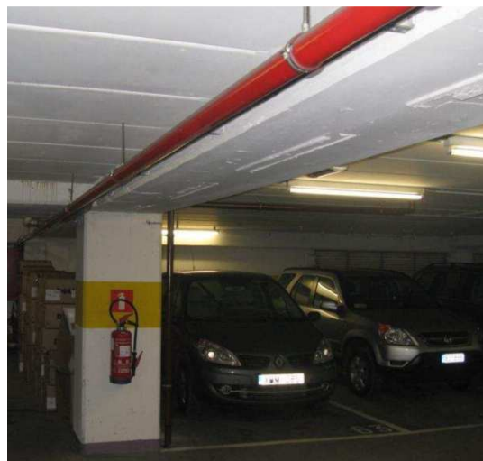
Figure 10: Parking fire safety piping network
