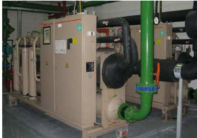
Figure 15: Water-cooled chilling package
