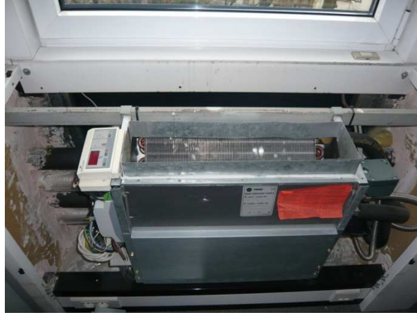
Figure 12: Concealed vertical fan coil unit
