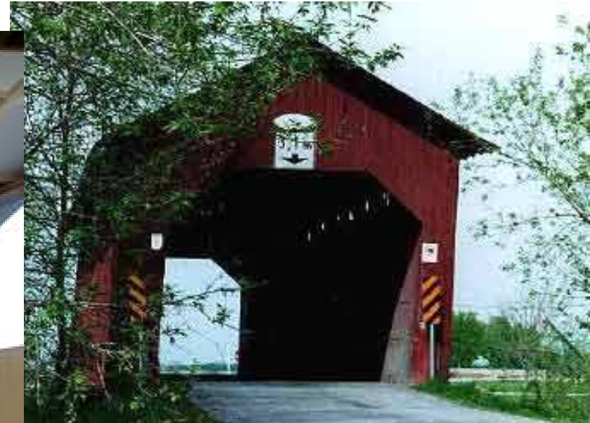
Pont couvert ND-de-Stanbridge, QC, Canada
