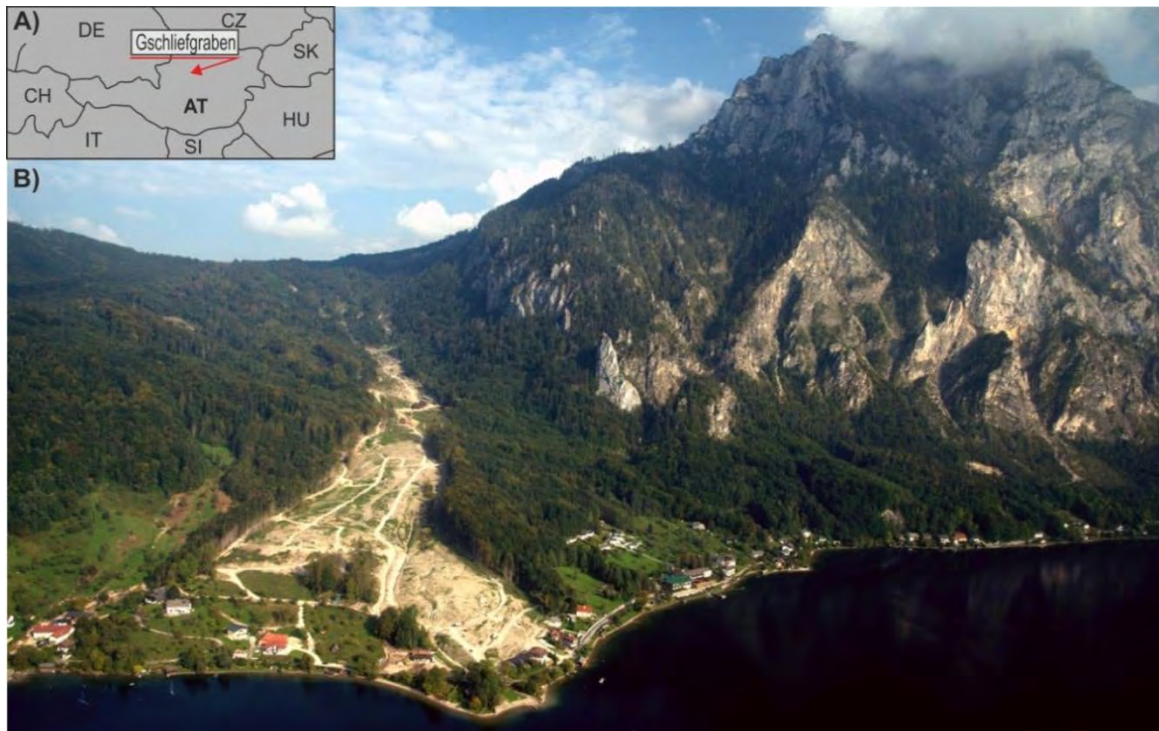
Fig. 1: General setting of the Gschliefgraben site: (A) Position within Austria, (B) Airborne photo of the Gschliefgraben valley and Mt. Traunstein from the west (Photo by: R. Supper, 2009).
