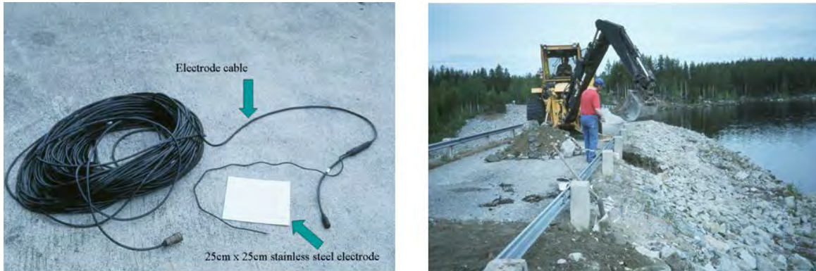
Fig. 1: Design of electrodes used for permanent installations for geoelectrical monitoring and photo from field installation in progress on Hällby embankment dam 1996.
