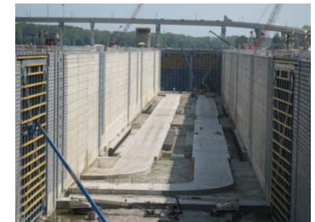
Fig 2: In-chamber longitudinal culverts, McAlpine Lock
