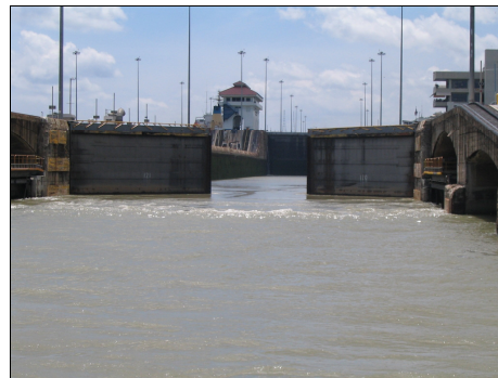
Figure 1 : Opening of gates (Miraflores) and density current at surface
