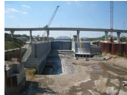
Fig 1: Intakes at new McAlpine Lock during construction
