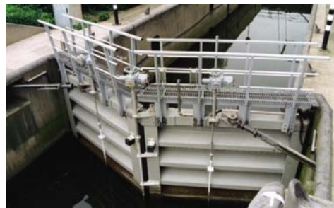
Fig. 1. FRP gate of a lock near Werkendam
