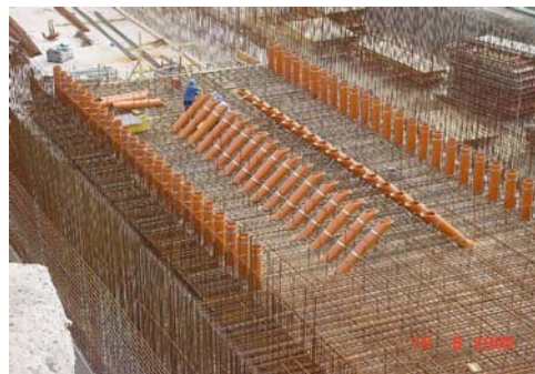
Picture 1: Permanent formwork for the pressure chamber of Sülzfeld lock
